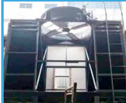
HDG Steel Structure
